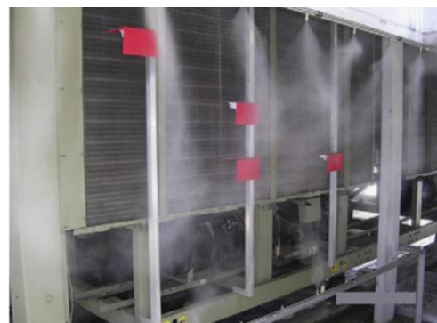
Fig. 14 (a) depicts A diagram illustrating the water vapor system, whereas (b) shows a snapshot with pertinent data.
